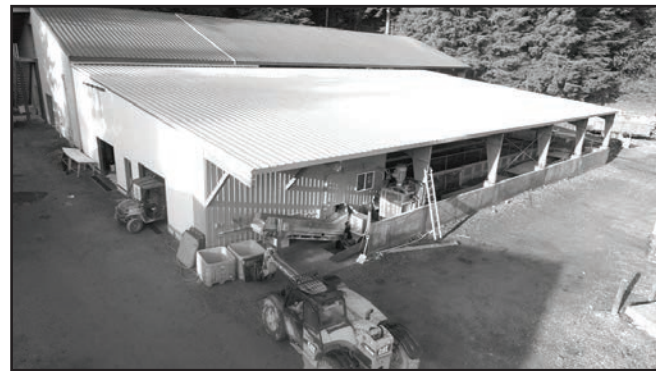
Hidden Falls spawning shed renovation nears completion.
