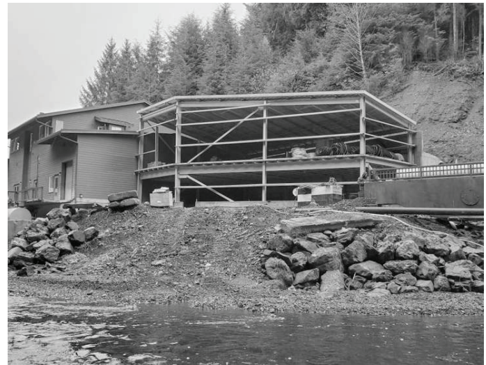
Construction continues at Gunnuk Creek Hatchery.
