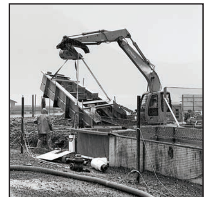
The fish ladder was removed.
