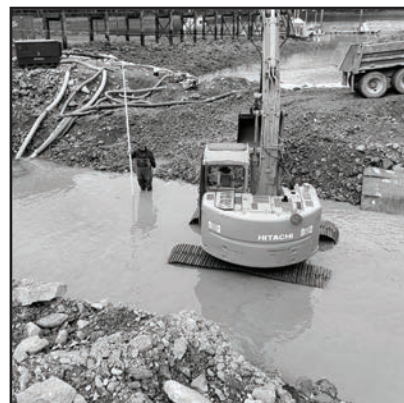
After the old log bulkhead was removed, the site was prepped for the new concrete panels.
