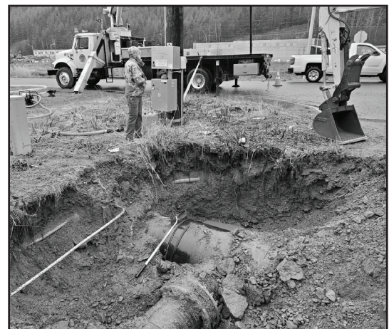
Bulk Line Repair at Sawmill Creek Hatchery
