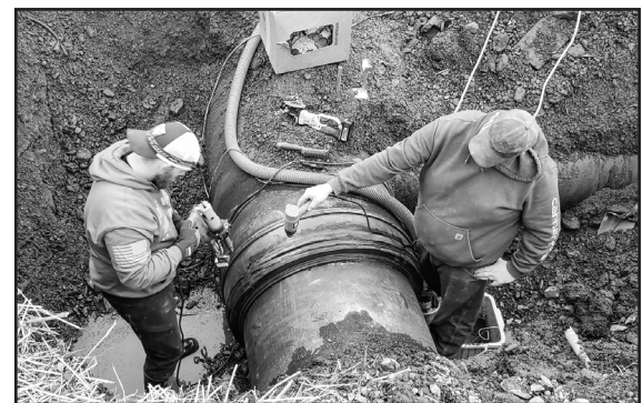
Cain DePriest and Kenny Gray weld HDPE pipe
