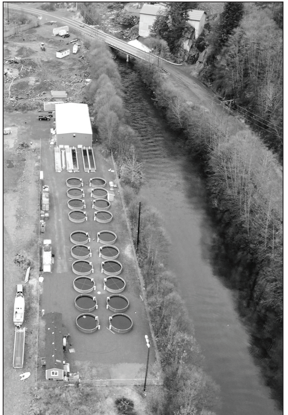
The expansion site next to Sawmill Creek Hatchery
