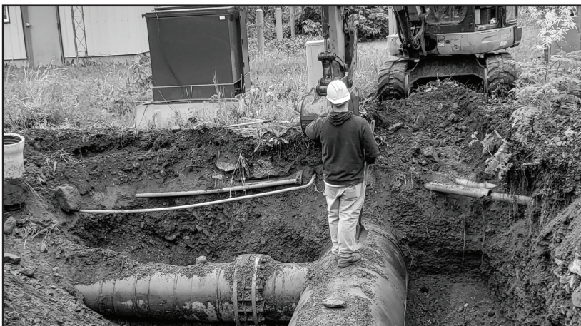
Bulk line construction at Sawmill Creek Hatchery
